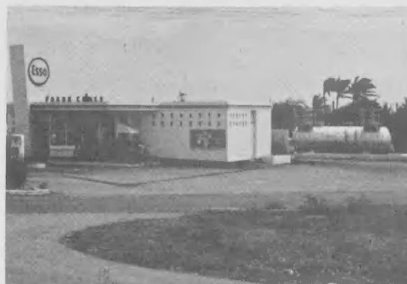
NEW GASOLINE tank for the Seroe Colorado Esso Station stands high and dry behind the building (left). The tank is divided in two sections, one for regular gasoline and one for Esso Extra (right).
